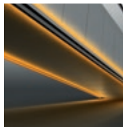
Side and soffit cladding*
