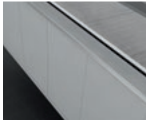
Grey powder coated sheet steel cladding (RAL7036)
