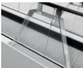
Anti-climb barrier (EN115-1:2008 + A1:2010 requirement)
