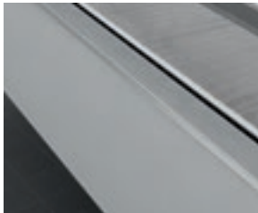
Grey primed sheet steel cladding (RAL7036)
